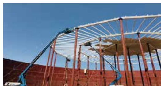
Girder & Rafter installation
