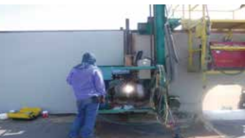
shell auto vertical welding
